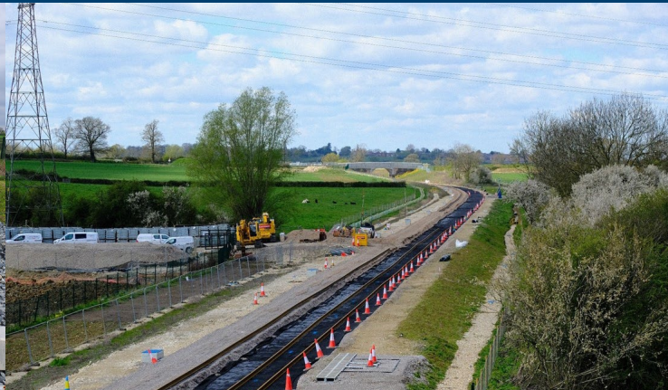
Rails ready for NTC at Verney Junction
