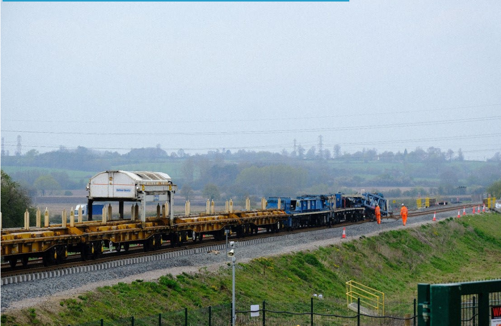
New Track Construction Train (NTC) in Winslow
