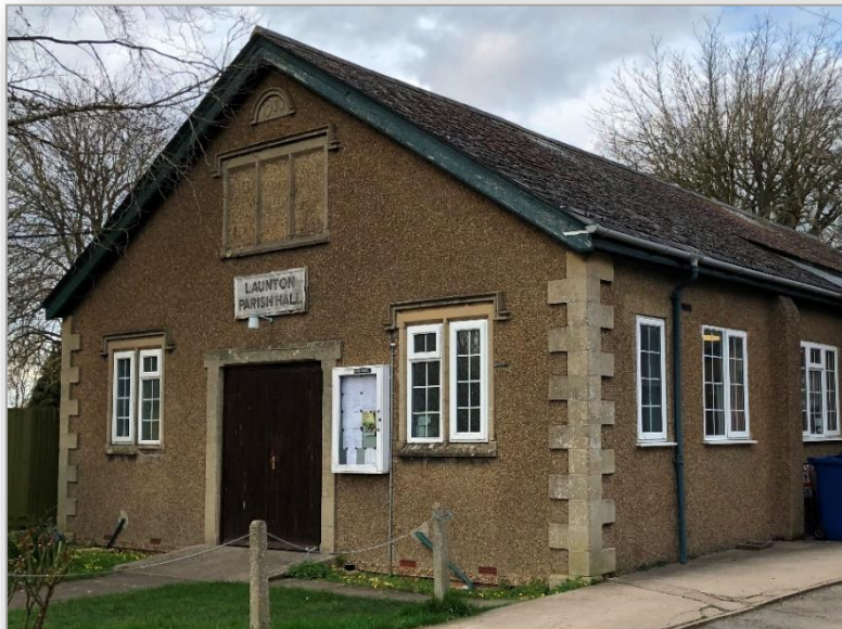
Current building detail, showing pebble dash elevations, moulded concrete window headers and sills, and moulded concrete quoins to front corners
