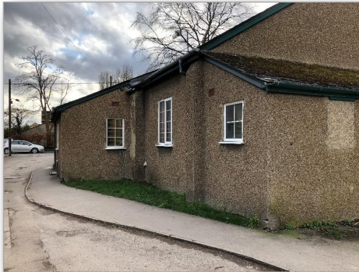
Launton Parish Hall: View of Side (Kitchen) and Rear (store rooms)
