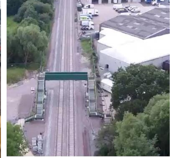
Bicester Fringe Commissioning London Road Level Crossing
