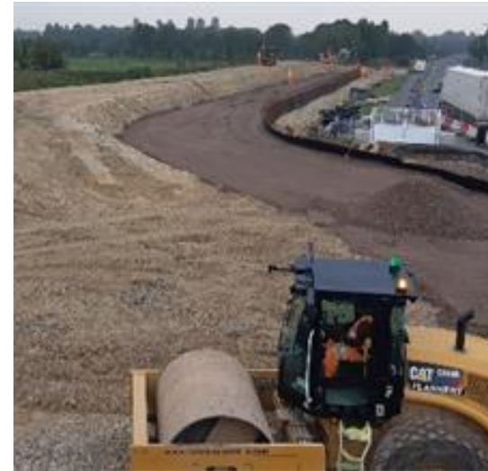
Charbridge Lane Traffic Switch
