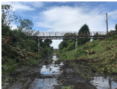
Site clearance in the Winslow Cutting
